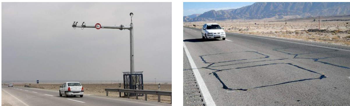
Figure 1. Photos of typical fixed speed cameras (left) and traffic counting inductive loop sensors (right) in Iran
