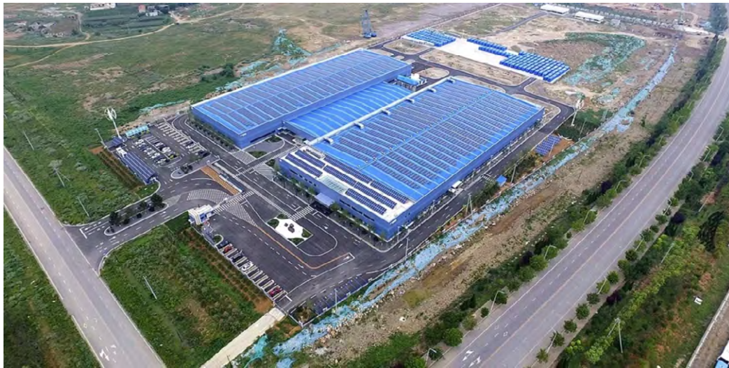
Figure 30. Redox Flow Battery Storage Demonstration Project
