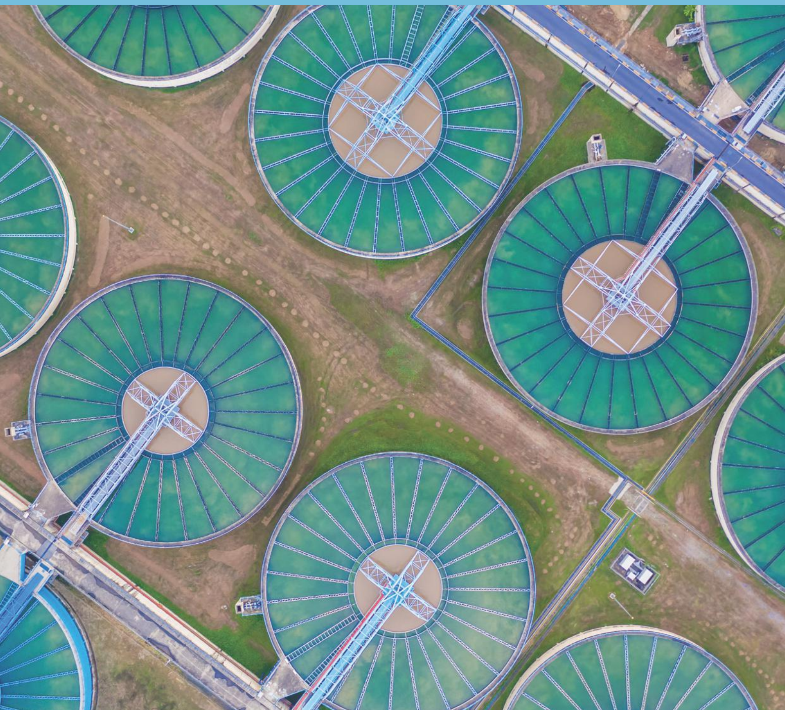
Aerial view of a water treatment plant.
