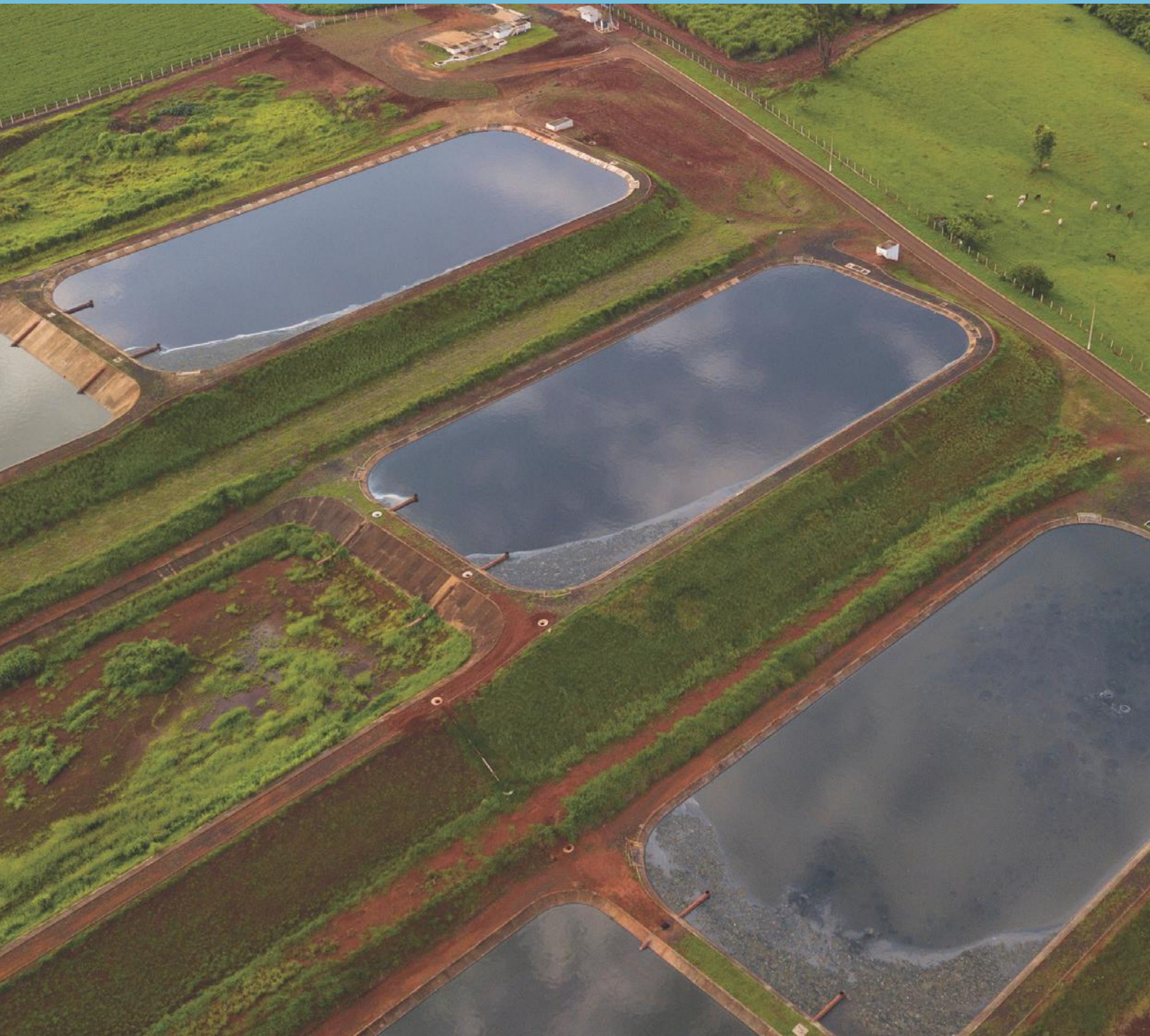
Aerial view of a sewage treatment facility.
