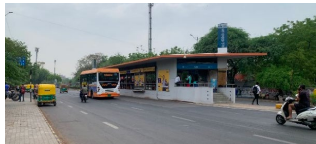
Level 2 – Transit operations in mixed traffic with priority at stations (Travel speeds 18-20 km/h)
