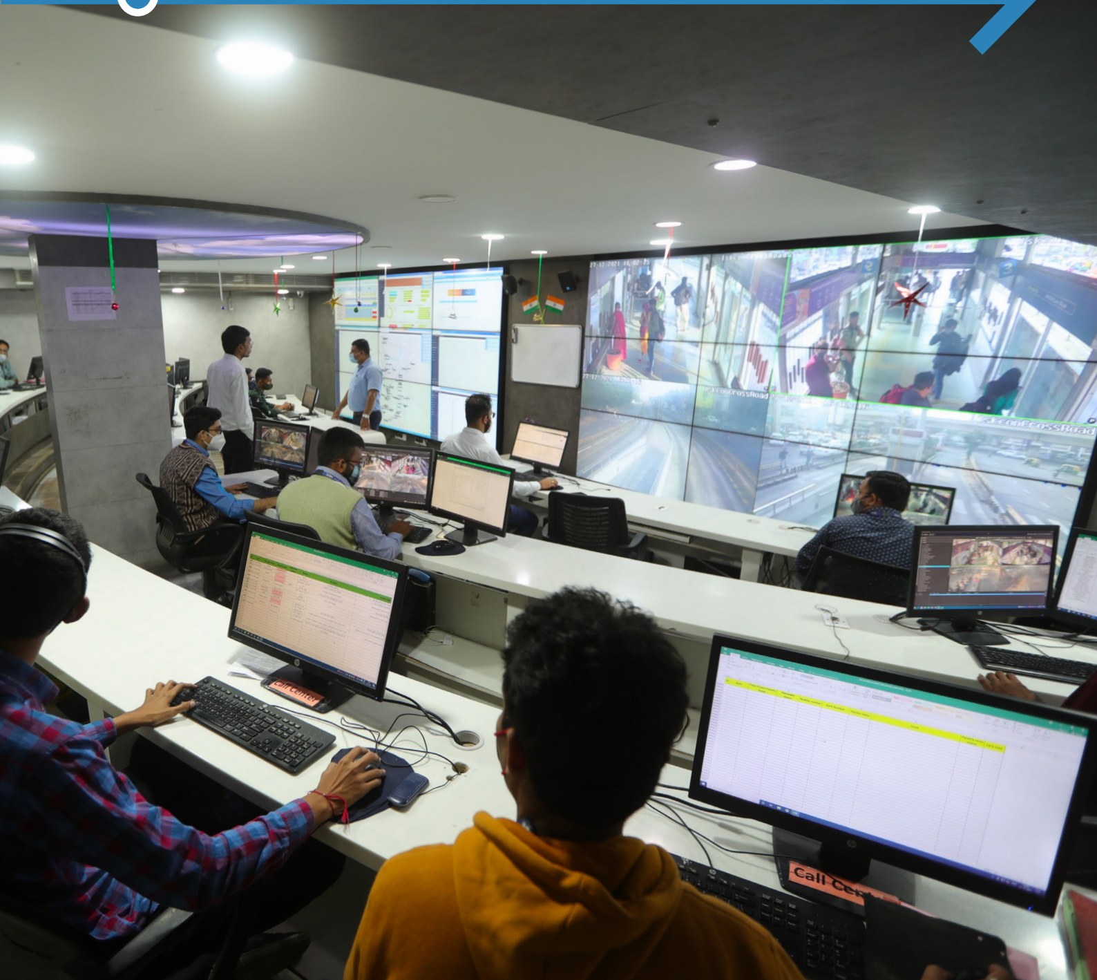
Command and control centre, Ahmedabad BRTS. Photo: CEPT
