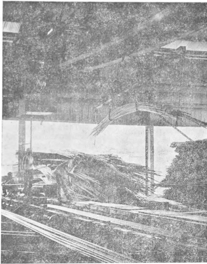
Workers stock steel rods, products of the National Iron and Steel Mills Ltd., the first major heavy industry to establish a plant on the Jurong Industrial Estate in Singapore.
