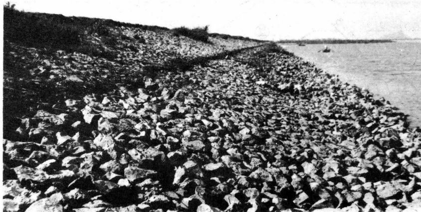
Figure 8. Armoured stone on seaside slope
