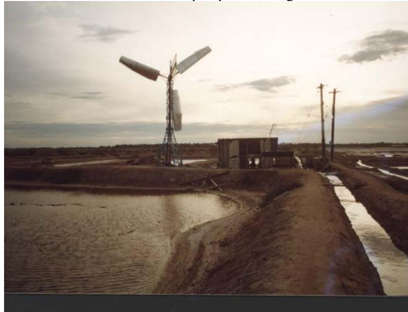
Figure 4.1 Water pumping windmill installed on the banks of salt pans
