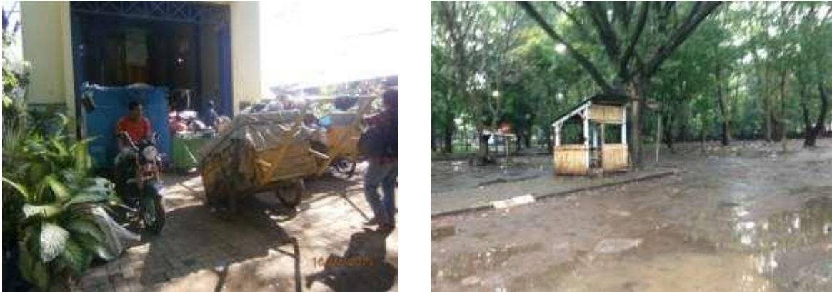
Figure 5 Velodrome Transfer Station
