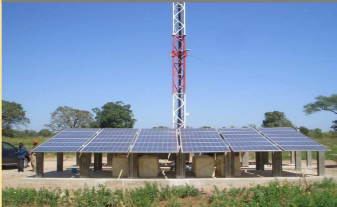
Figure 6: Solar station at a mobile network site in Senegal
