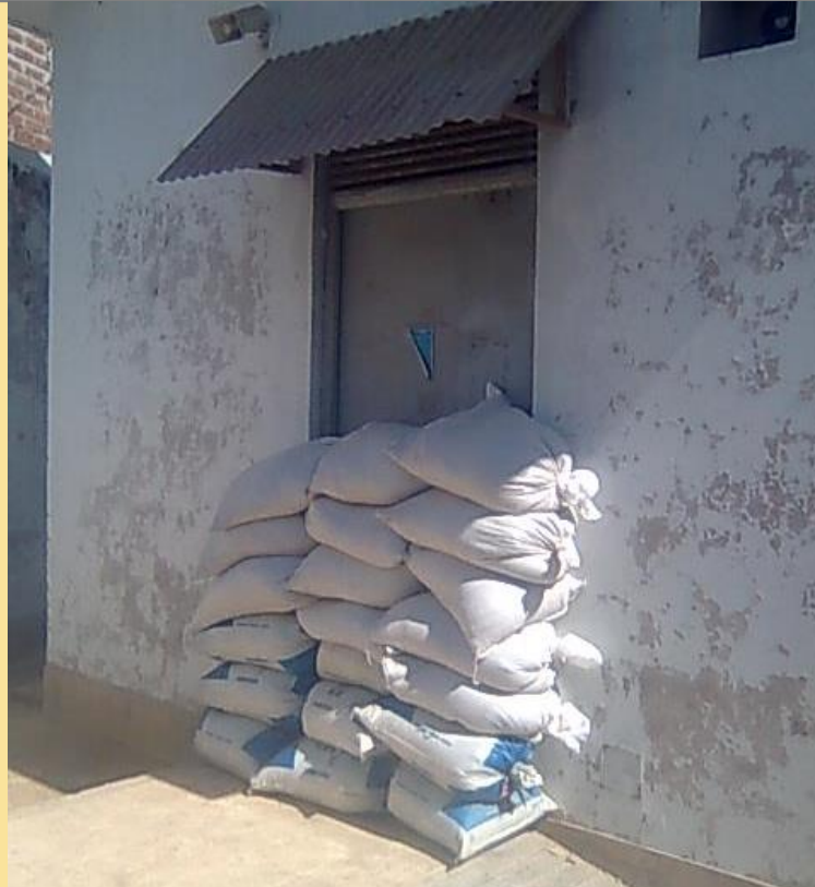
Figure 3: Locking the door with sandbags to prevent floodwater from affecting network sites
