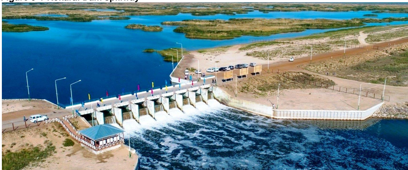
Figure 3-1 Kokaral Dam spillway
