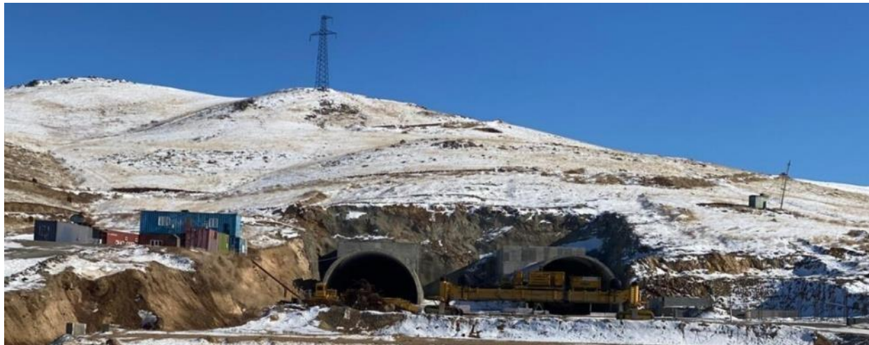
Figure 9. Construction of road tunnel in Turkestan oblast. 118
