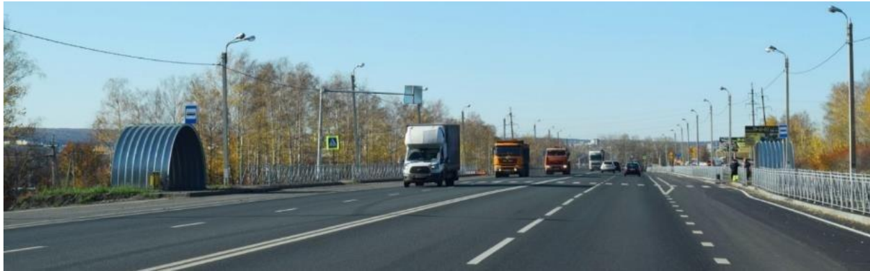
Figure 14. The M-5 “Ural” Orenburg-Moscow road bypassing a settlement.
