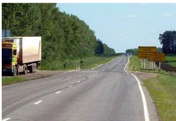
Figure 13. A typical view of P-239 road “Orenburg Highway” in Orenburg oblast.
