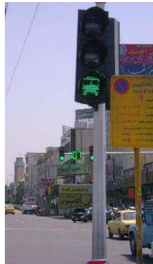
Figure 14 Real-time bus priority signal for late buses
