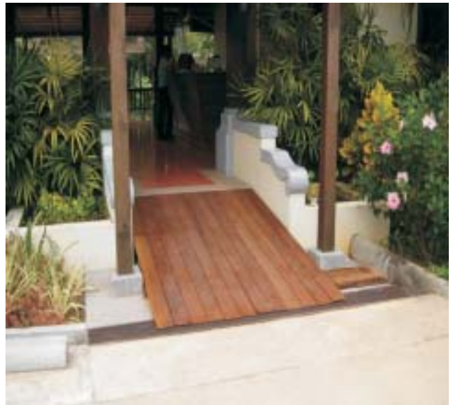
Post-disaster rebuilding presents opportunities to rebuild with universal access features. (Disabled People's International photo)
