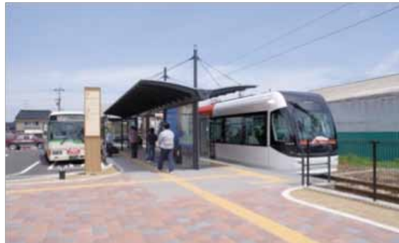
Japanese multi-modal station for bus and train in Toyama City (Iwasehama station)
