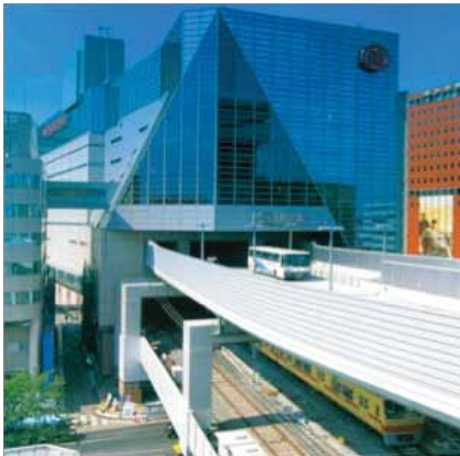
Japanese multi-modal stations: Nishitetsu Tenjin station in Fukuoka City in which the second floor is used as the railway station while the third floor is a bus terminal and the fourth floor is a parking area.
