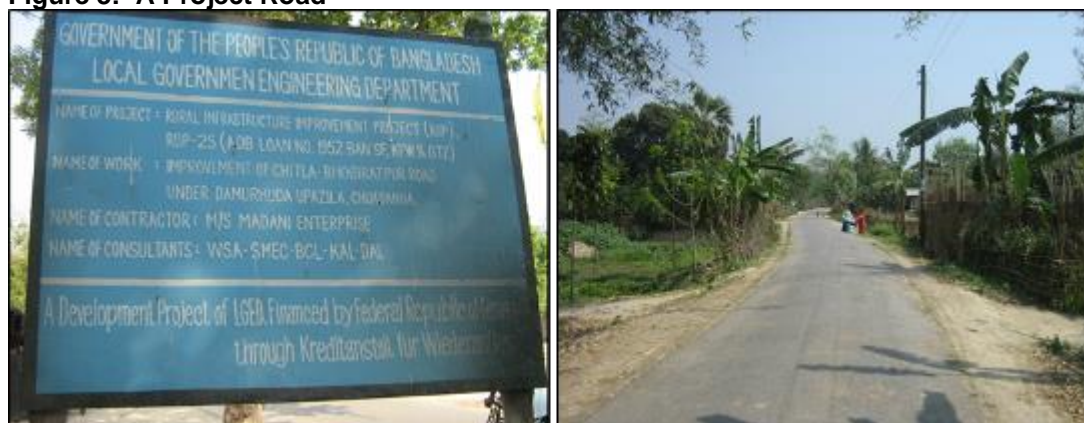
Figure 3: A Project Road
