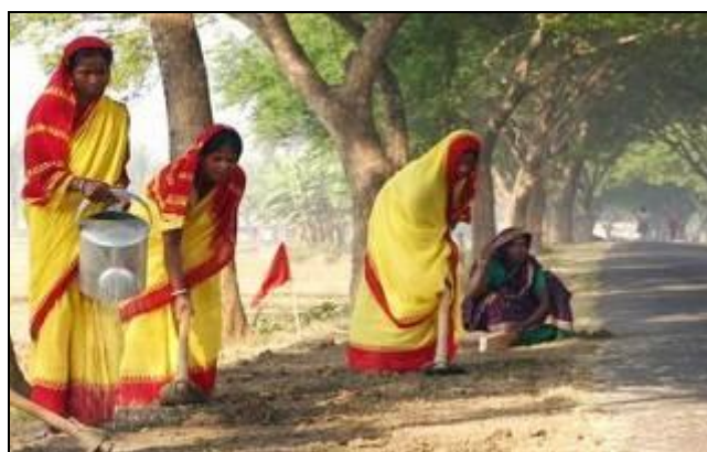
Figure 6: Female workers in construction works
