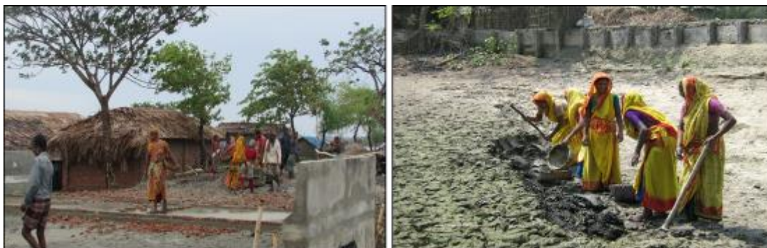
Figure 5: Female workers in construction works
