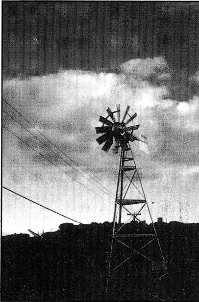
Windsparge cleaning a petroleum-contaminated site at North Ontario in Canada
