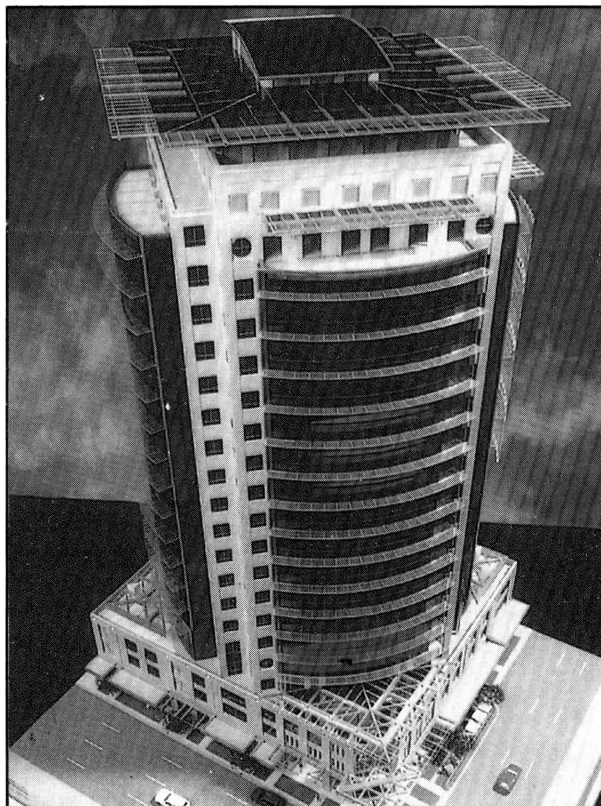
A model of the 80 kW integrated PV system
