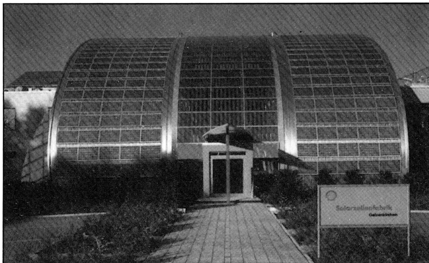
Shell's latest PV manufacturing plant in Germany
